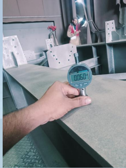
SA 2.5 Steel Shot/Grit Blasting
