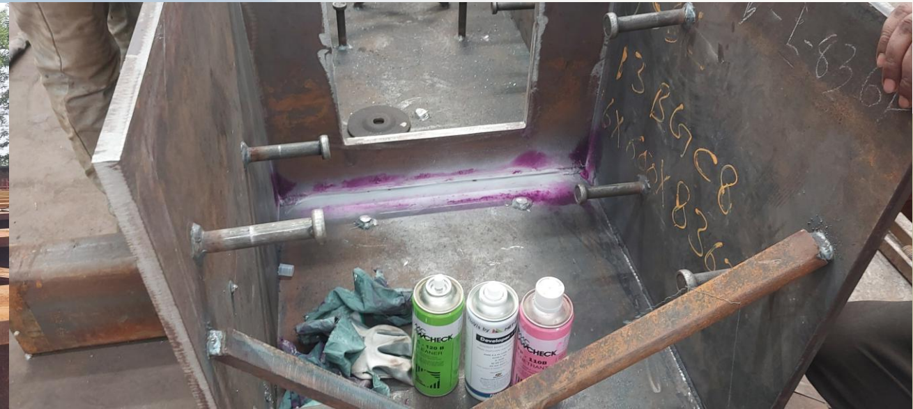
100 % DPT Testing on Weld Joints (CFW, PPBW, FPBW) . . .
