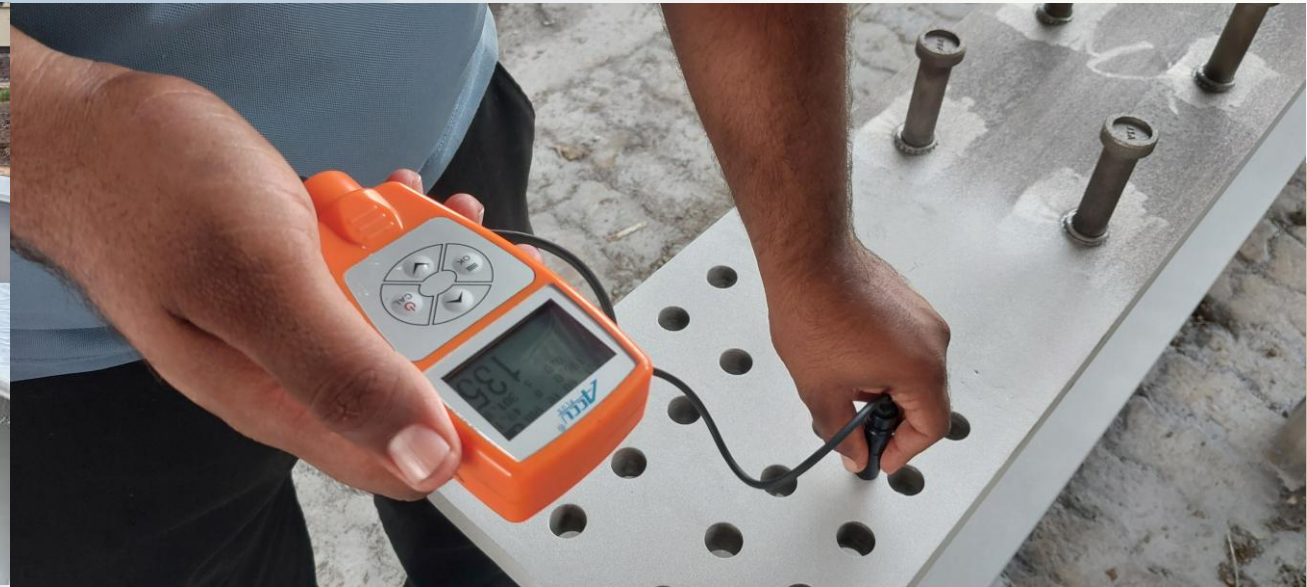
Dry Film Thickness (DFT) Checking
