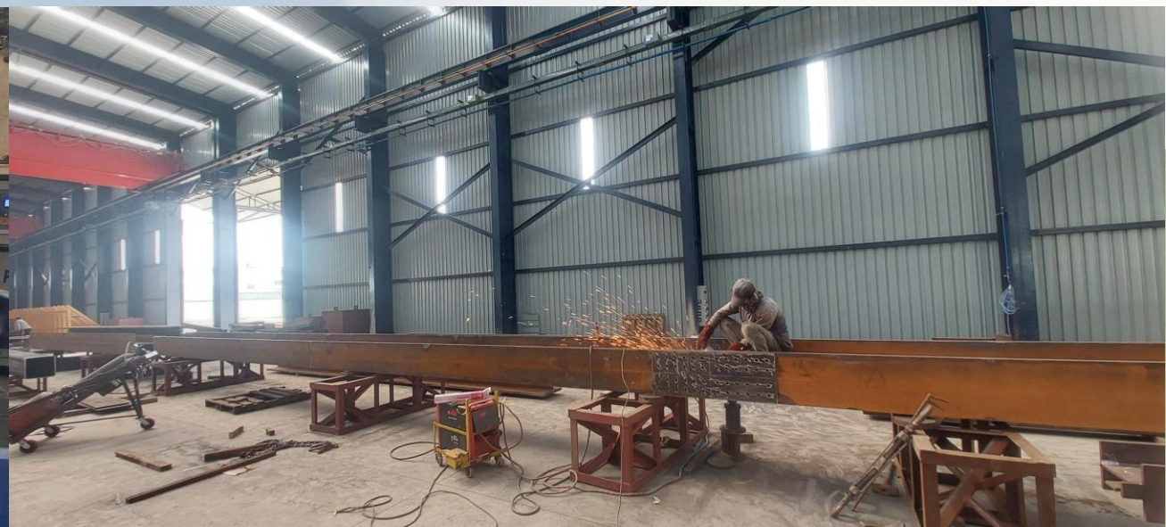
Girder Butting and Finishing
