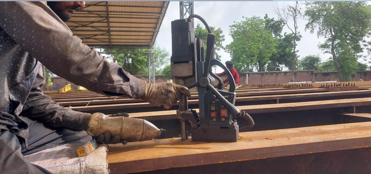
Magnetic Core Drilling on Flange/Web
